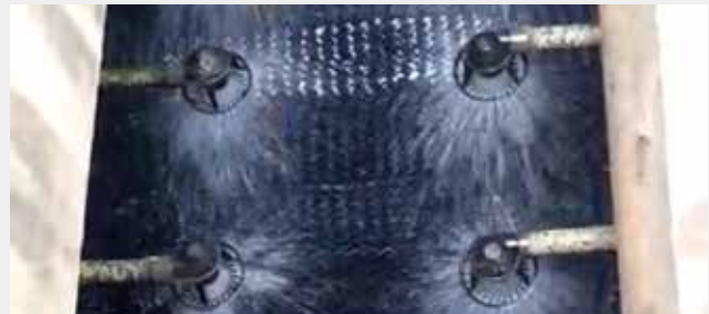
Before replacement of Nozzles
