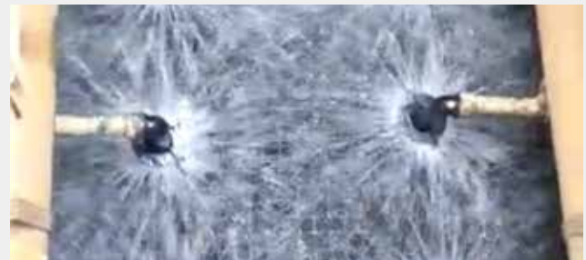
After replacement with energy efficient Nozzles
